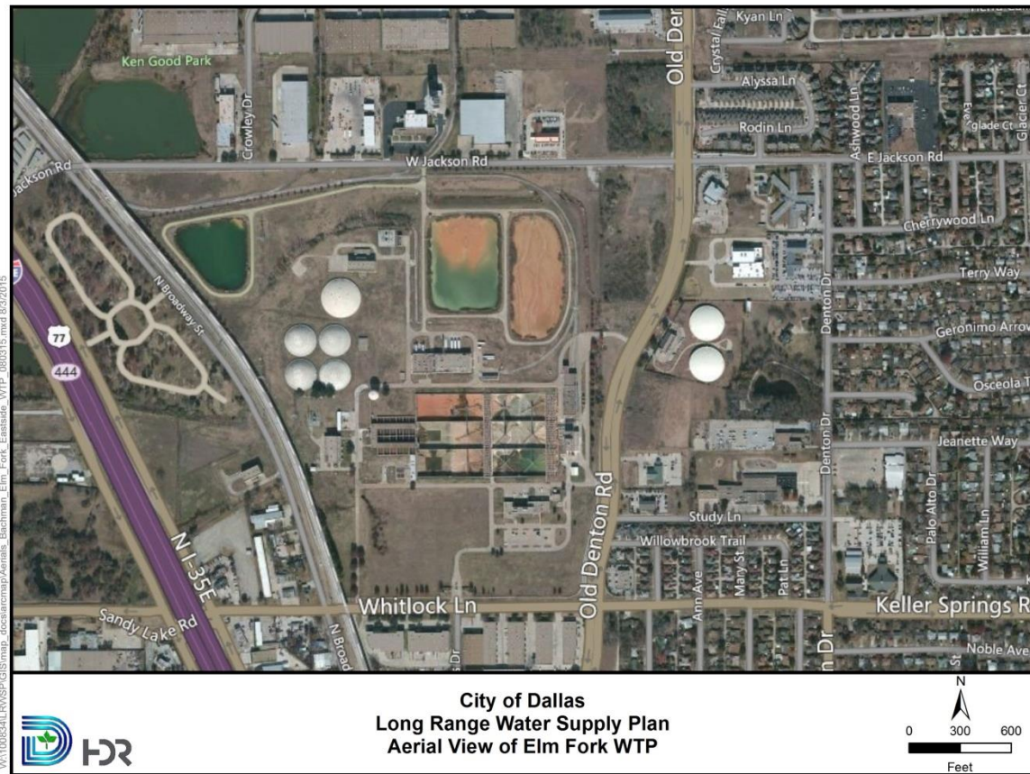
Figure 8-3. Aerial View of the Elm Fork WTP
