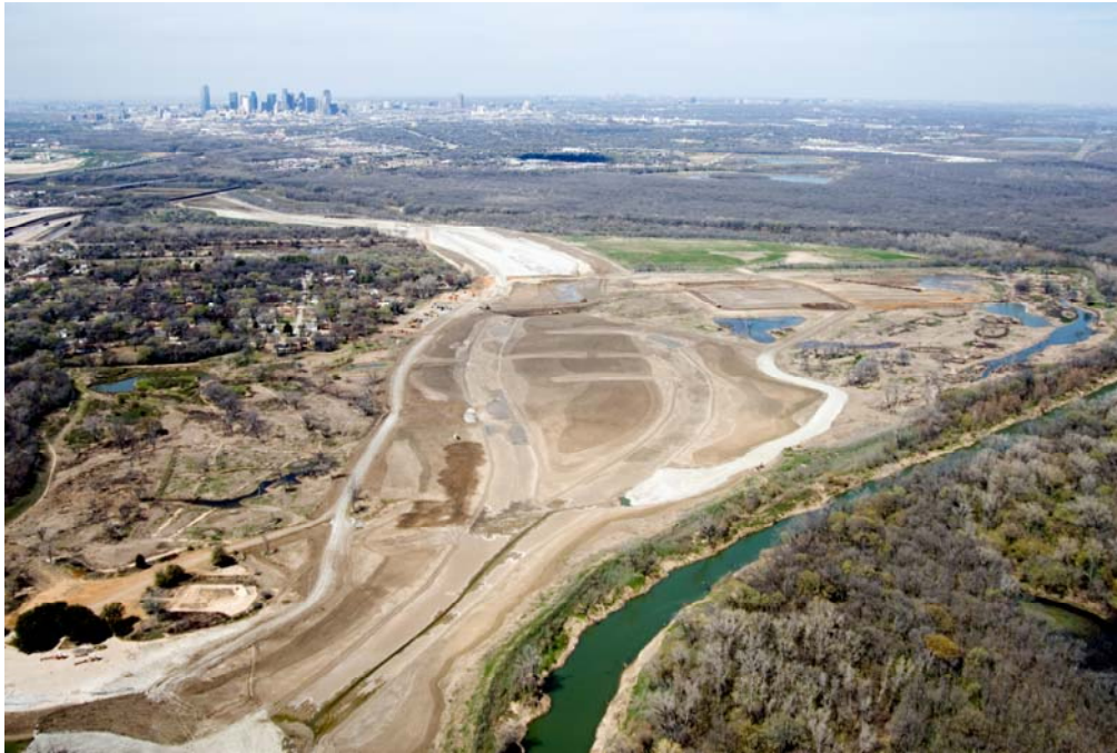
Cells E, F and G, looking north from Loop 12, into what used to be the Sleepy Hollow Golf Course
