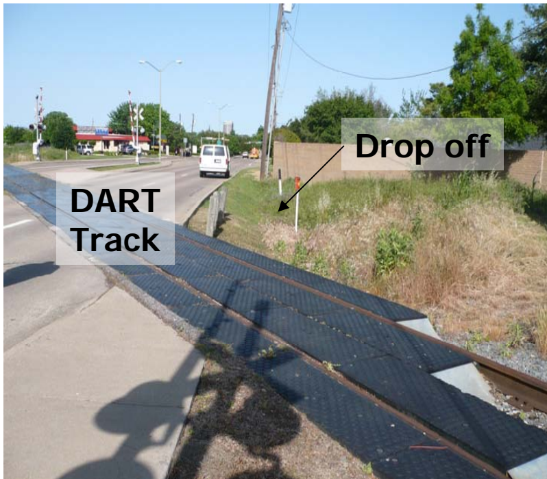
RR track crossing Complicated due to RR involvement and slope Location: McCallum Blvd.
