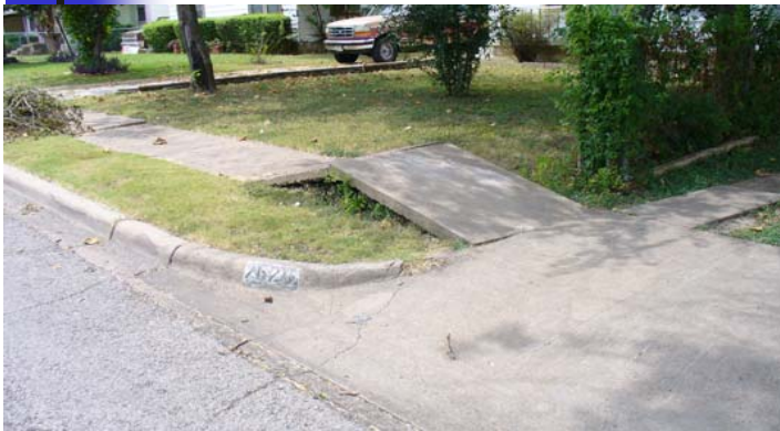
Location: Overton Rd
