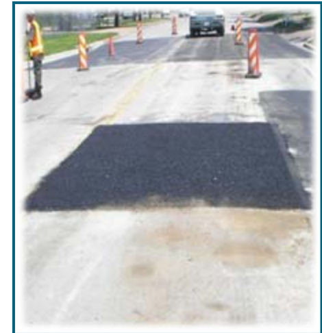
Full-Depth Asphalt Repair
