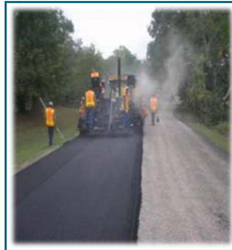
Rehab/Restoration Overlay
