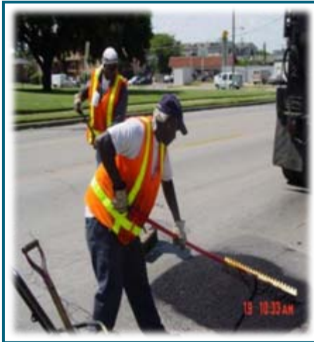
Pothole Repair
