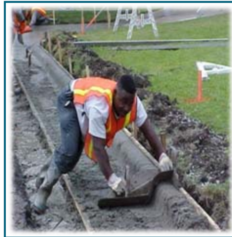
Curb and Gutter
