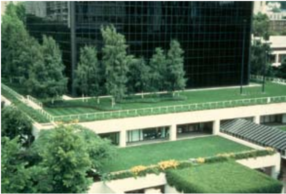
Eco-roofs reduce storm water run-off from roofs and offer pleasant landscaping for building tenants. Vegetated roof treatments help cool the building in the summer and provide added insulation in the winter.
