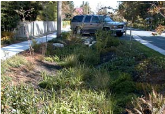
A neighborhood bioswale absorbs water run-off and filters road and parking pollutants on-site utilizing principles of storm water management.
