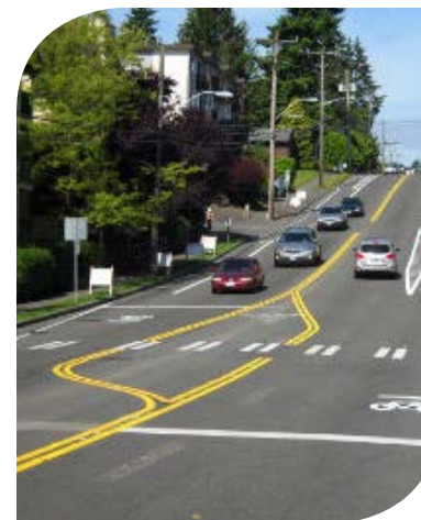
Bike lane and buffer transition at intersections
