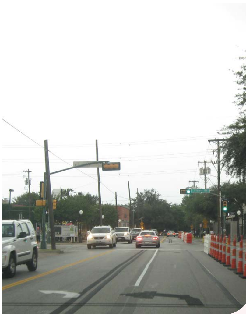
The Knox Street demonstration used blackout tape to temporarily cover up existing pavement markings.
