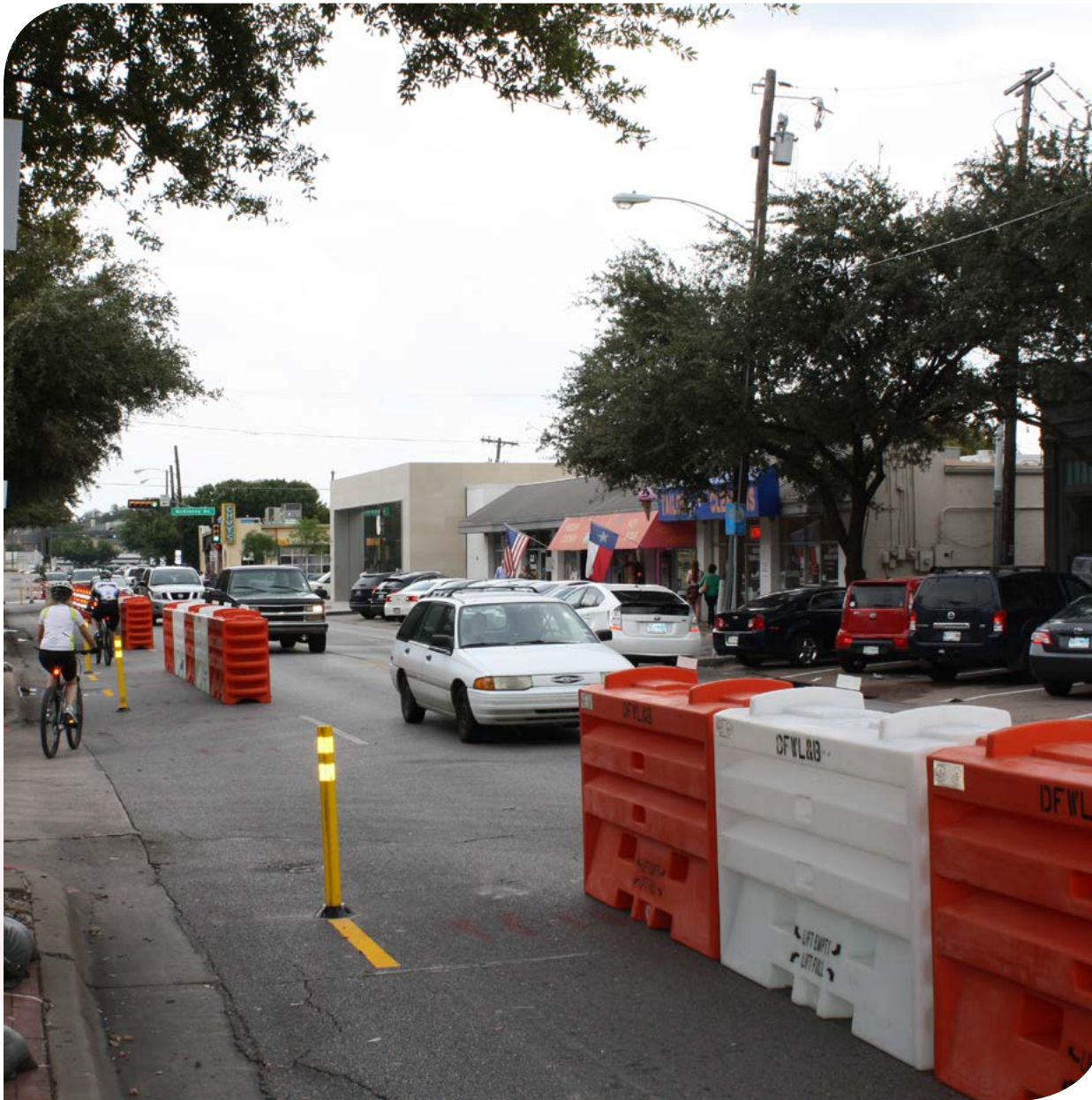
The Knox Street demonstration tested the installation of an eight-foot cycle track.
