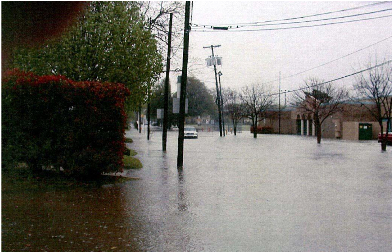
Worth Street Flooding
