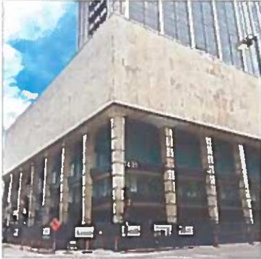
94% of the historic marble is removed. THC / NPS approved the refurbished marble mock installation (seen on the 3<sup>rd</sup> from right column crown)
