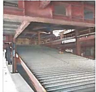
Floor cutouts were made and new steel ramps are installed from the street level to the added parking garage on fl. 6-8 (behind the windowless marble façade)
