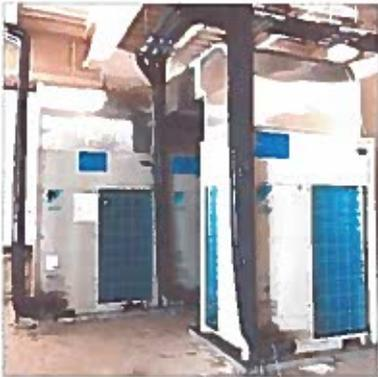
**28 high energy efficient VRV HVAC units are installed**
