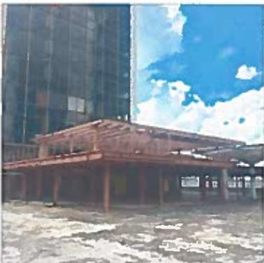
New steel structure is installed for restaurants and bars on the 75,000 sq.ft. amenity deck
