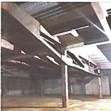
New structural support steel was fabricated and it is installed on levels 6-7 (pictured level 6)
