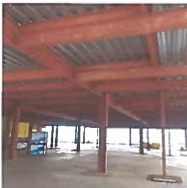
New steel structure installed on fl. 9 (amenity deck) & 10 (above)
