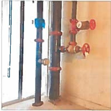
**Four (4) fire sprinkler standpipes are installed (standpipe pictured in west-end staircase)**
