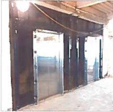
**Elevator openings were cleared and new frames, sills and doors are installed on 15 floors**
