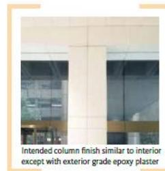
Intended column finish similar to interior except with exterior grade epoxy plaster
