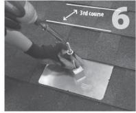
Slide flashing into position. Prepare hanger bolt with hex nut and sealing washer. Insert into hole and drive hanger bolt until QBlock stops rotating easily. **Do NOT over torque**.
