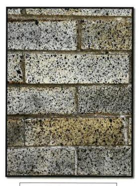
Existing brick was treated with a form of acid or wash to change color
