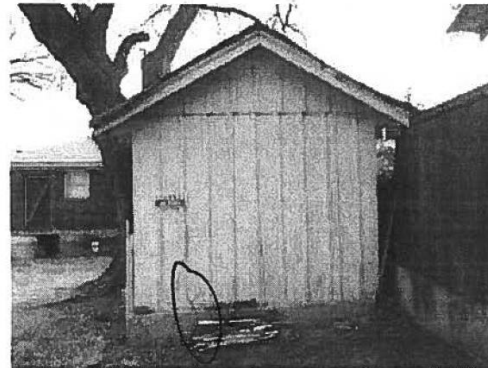
North side. Note the fractured concrete
