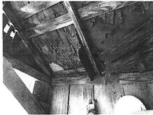
Rotted wood shingles and sheathing.
