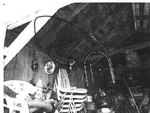
Severe rot to roof structure. Noet the
