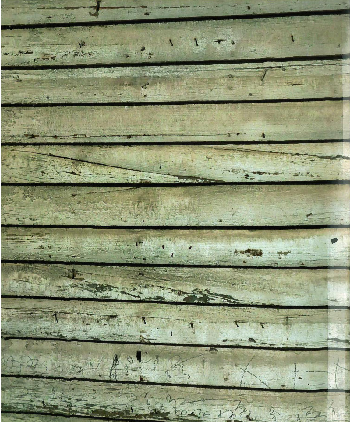
Existing siding on main structure with 4" exposure.
