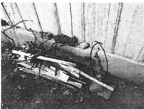
Fractured Curb
