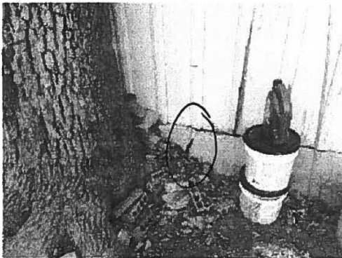
Fractured concrete curb on the east side.
