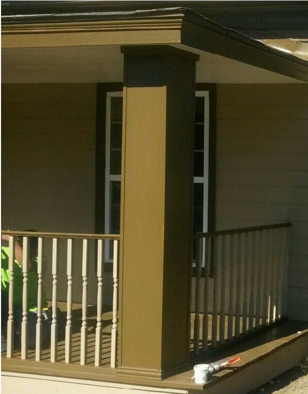
Requests #3 & #4: Porch railing and columns as installed.
