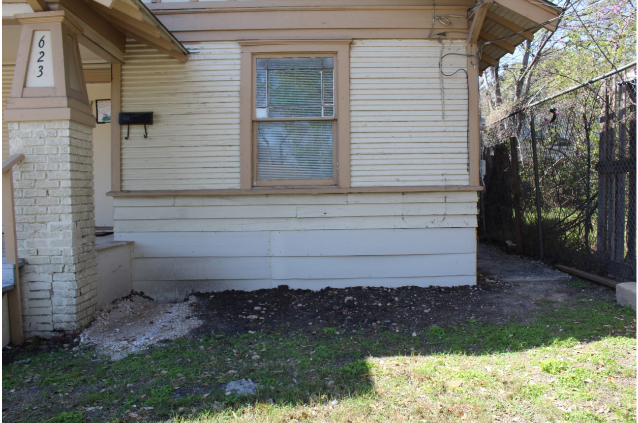
Front elevation detail. Note: wood has been used as a temporary fix to enclose the foundation of the structure.
