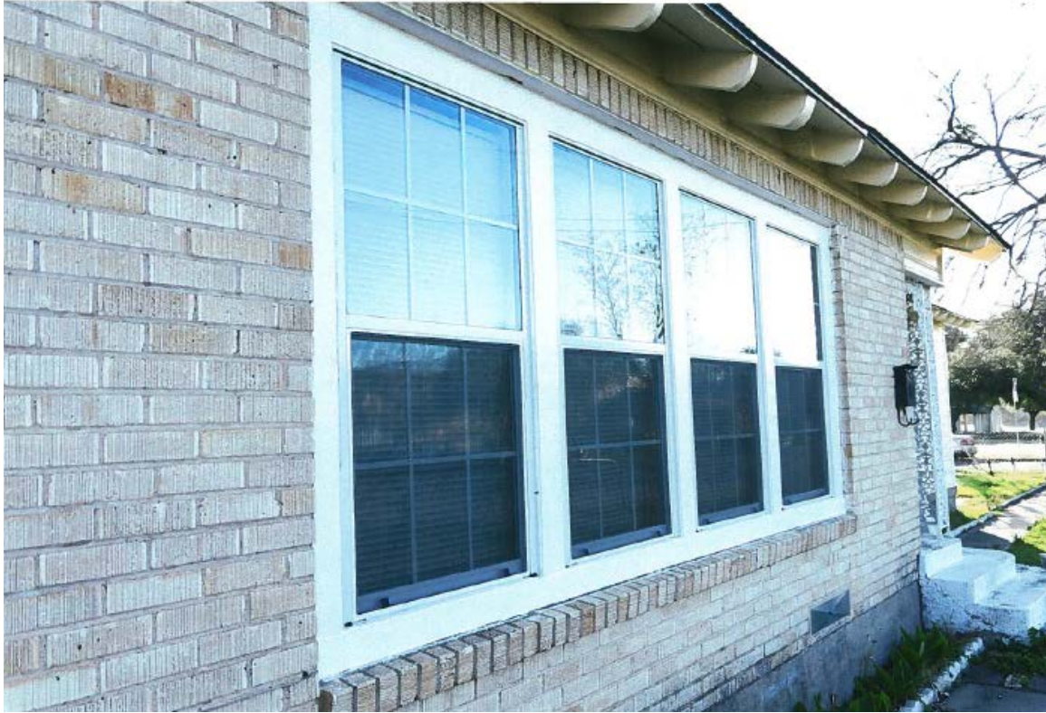
Close up of four new aluminum windows on left side elevation, photo submitted by applicant.
