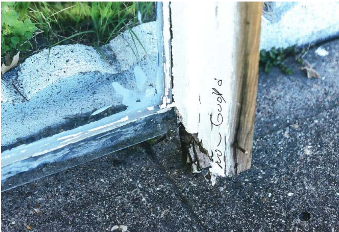
Photo showing window deterioration, submitted by applicant.
