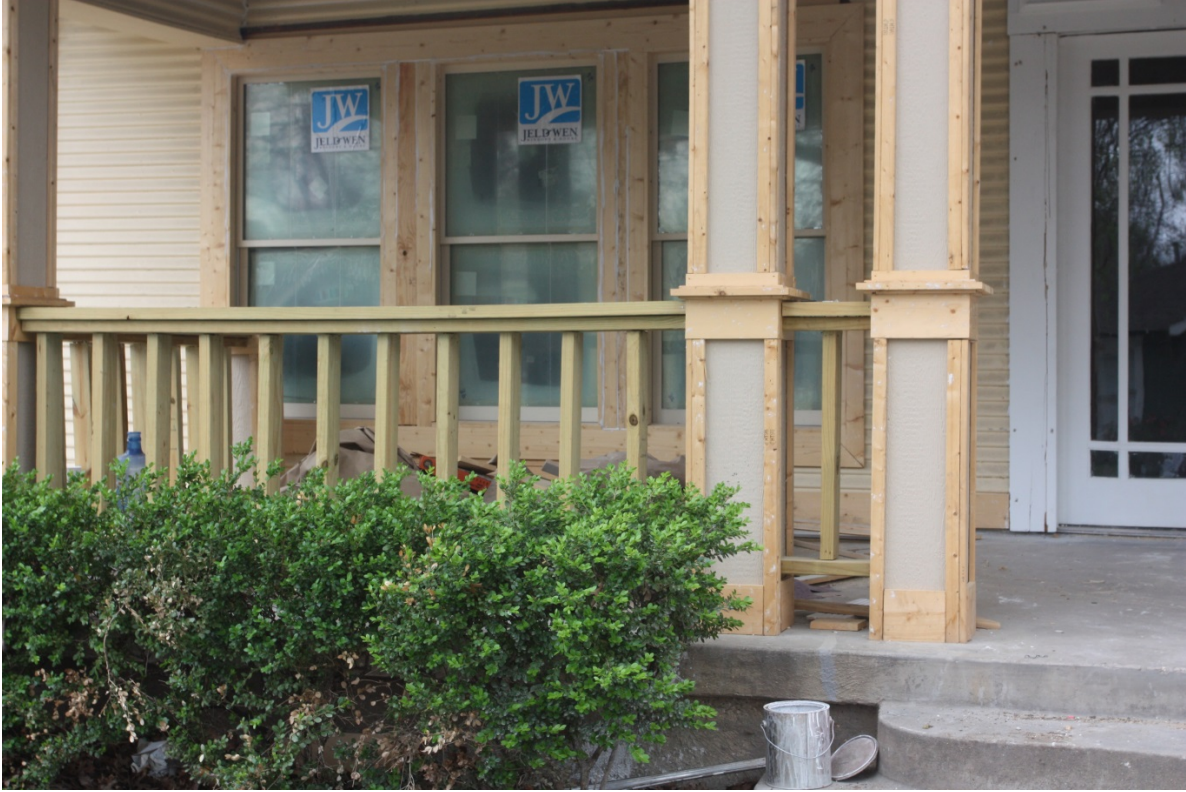
Close up of initiated work on columns and rails, left side of front elevation.
