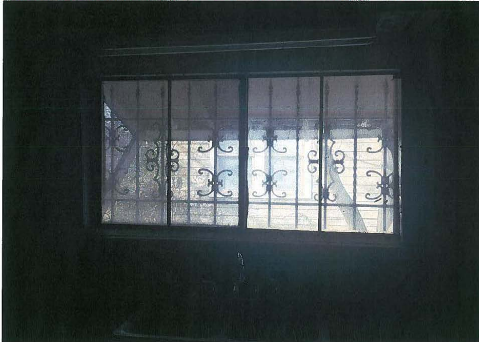
REPLACE WITH PAIR OF 2'-4" X 2'-10" WOOD WINDOWS
