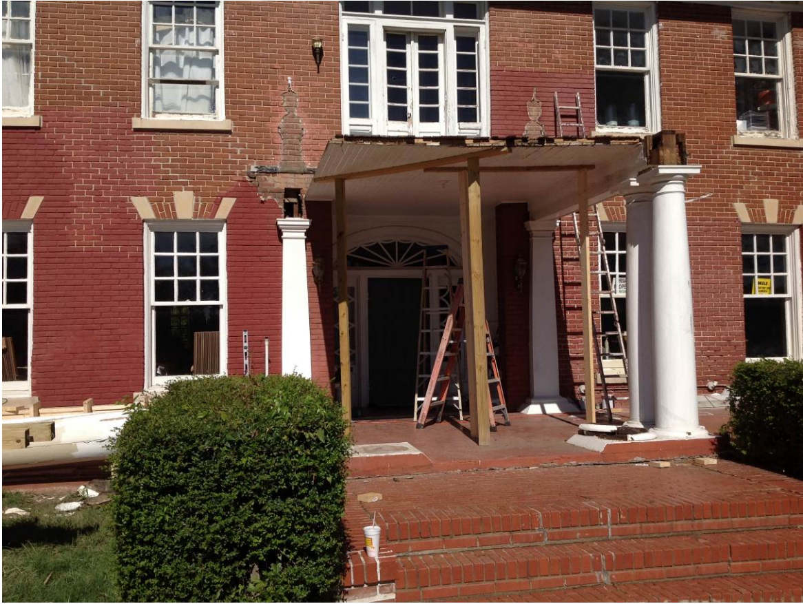
Photo from 2013, showing problems with brick repointing and attempts to cover with paint.
