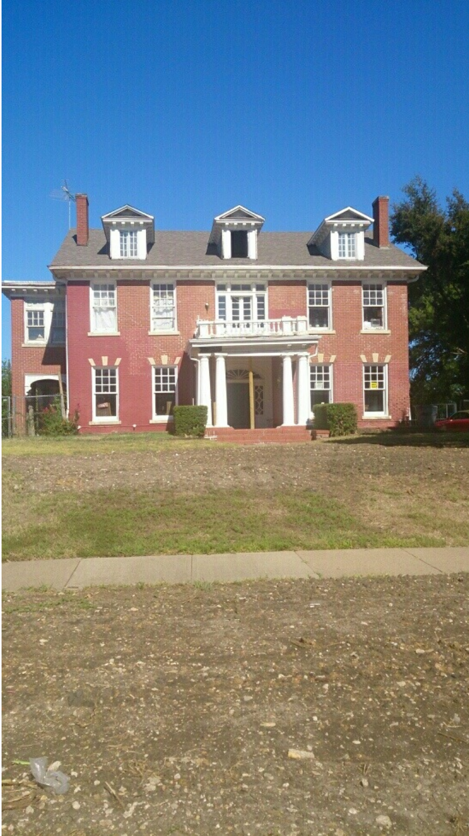
Photo from 2014, showing problems with brick repointing and attempts to cover with paint.
