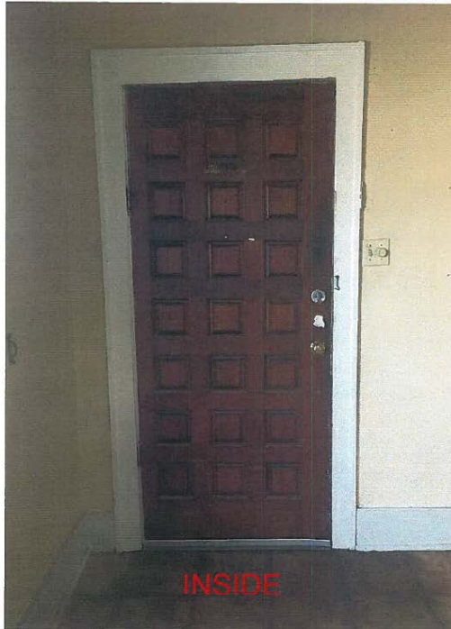
EXISTING FRONT MAIN ENTRY DOOR - 2'-10" X 6'-8"
