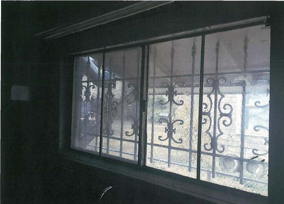
REPLACE WITH PAIR OF 2'-4" X 2'-10" WOOD WINDOWS
