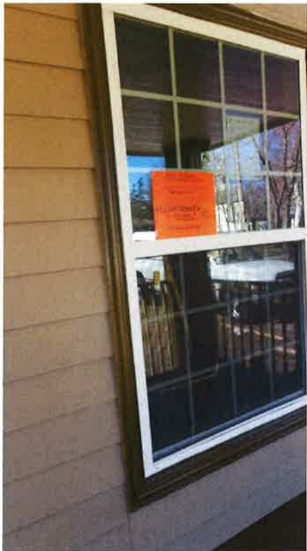
Close-up of installed windows – SDL, flush mounted, sills and original trim also removed
