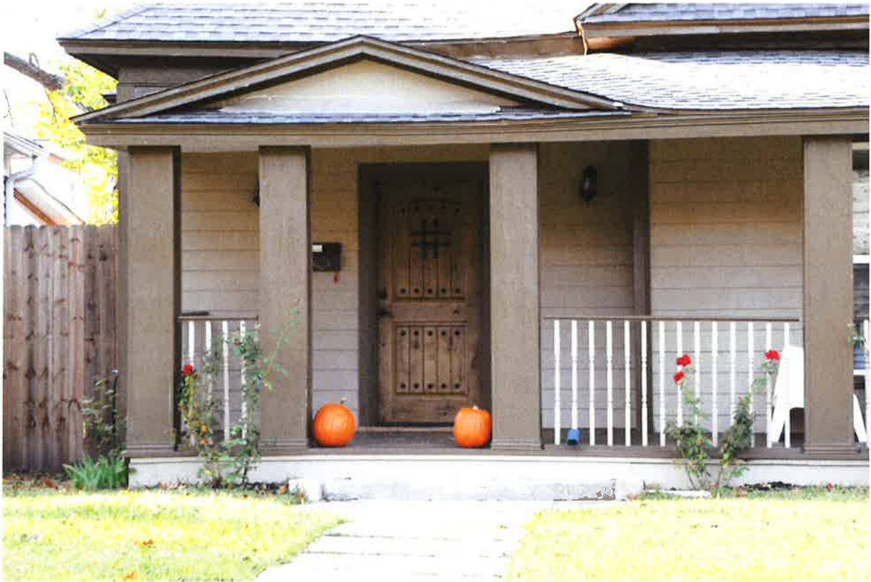
Installed new door
