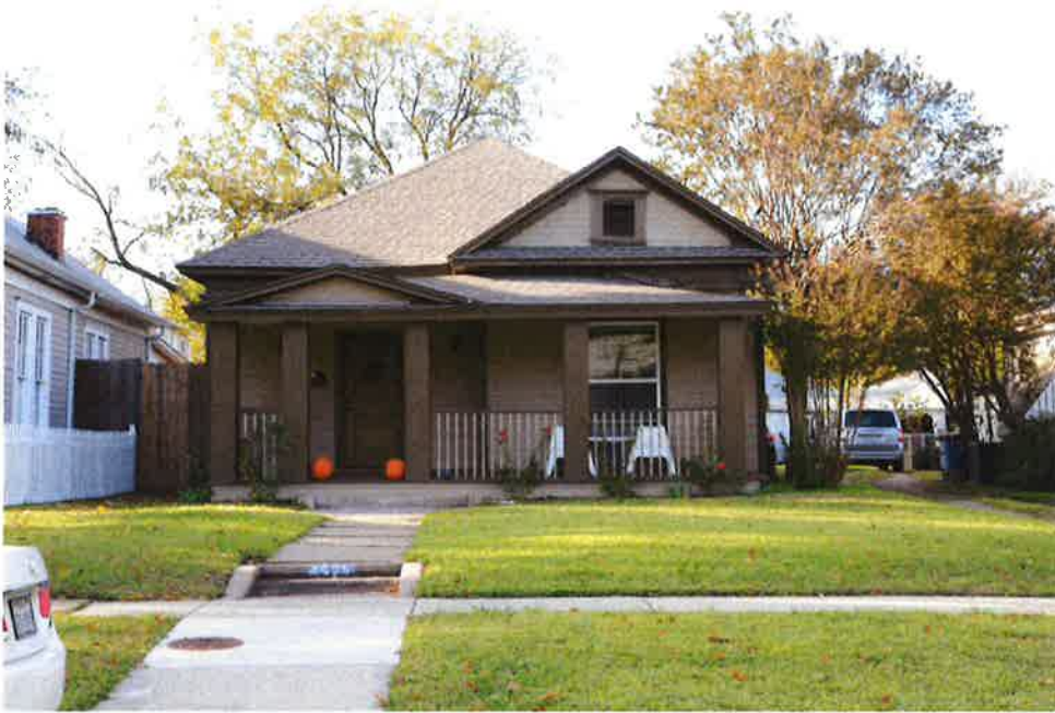
Current front porch column configuration
