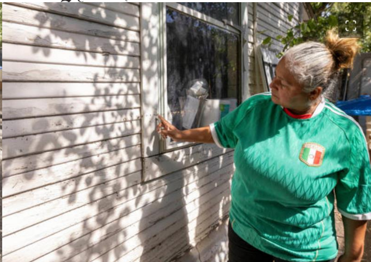
Gloria Alvarez points to the flood water line on the outside of her home along Alcalde Street. Several homes along Alcalde Street were flooded on Aug. 22, including Alvarez.
