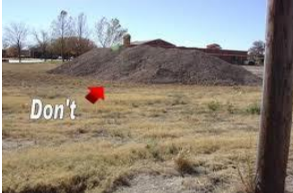
Figure 1 Stockpile exposed to weather
