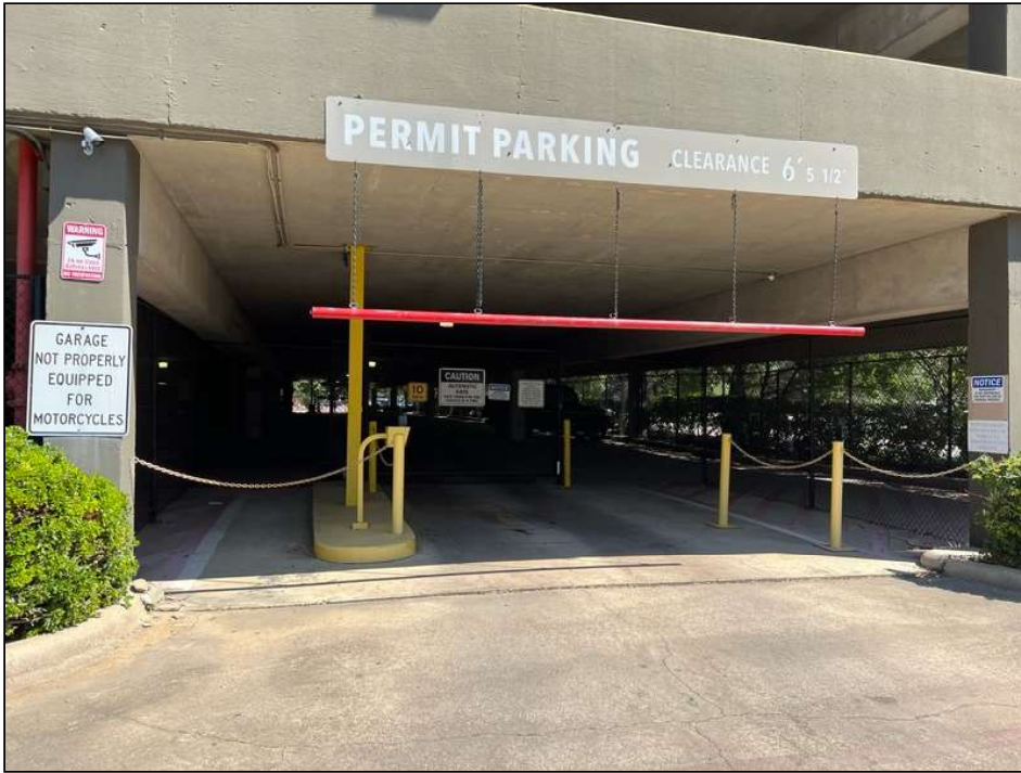
11. Secure access at parking garage
