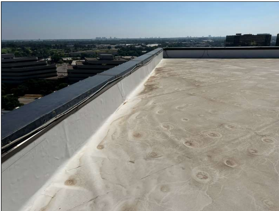
16. Roof parapet and membrane condition
