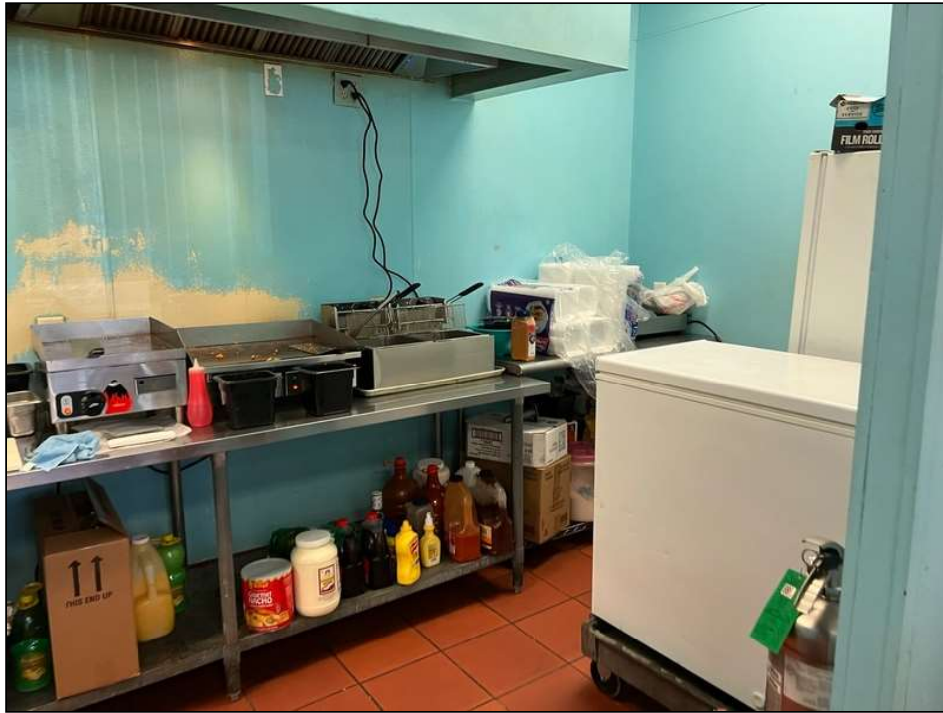
67. Ground floor Deli finishes
