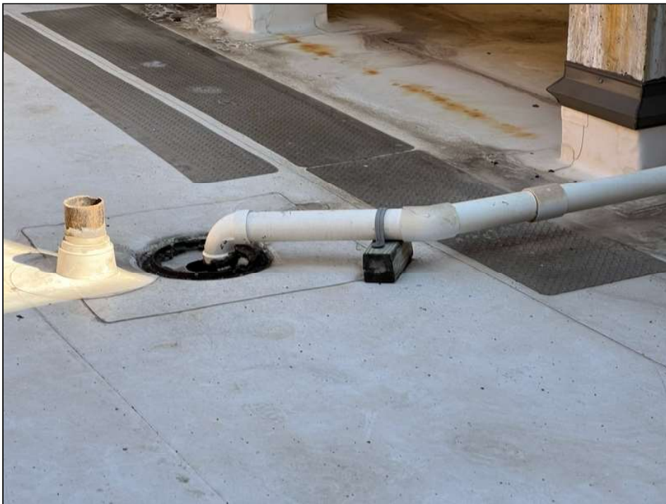
14. Interior roof drain
