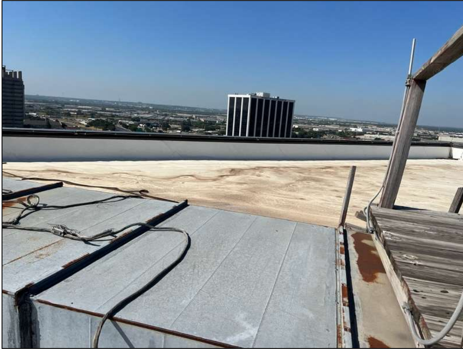
13. Low-sloped TPO roofing
