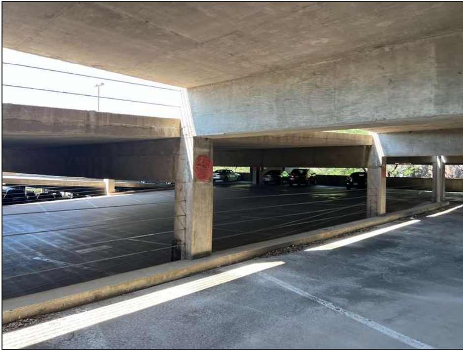
75. Parking garage concrete structure
