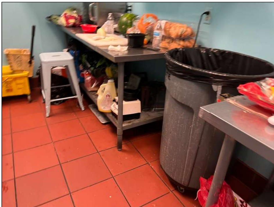
68. Ground floor Deli finishes
