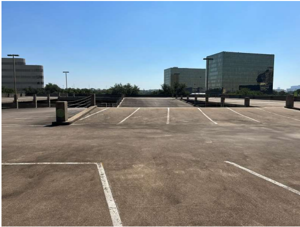
Parking garage concrete structure
