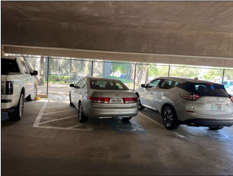
81. Missing accessible parking signs
