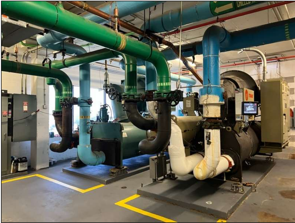
21. Domestic water piping
