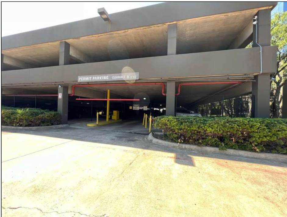
10. Secure access at parking garage
