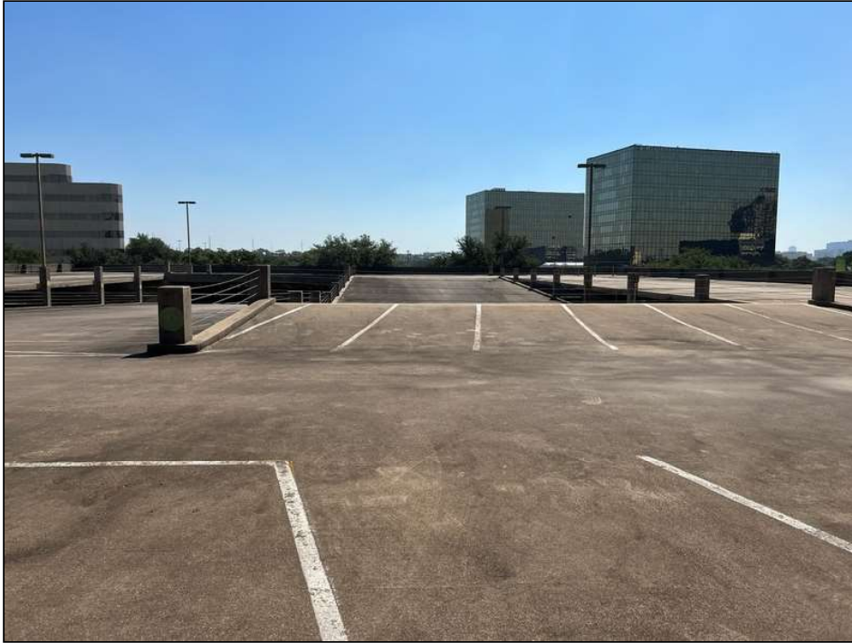
9. Parking garage concrete structure
