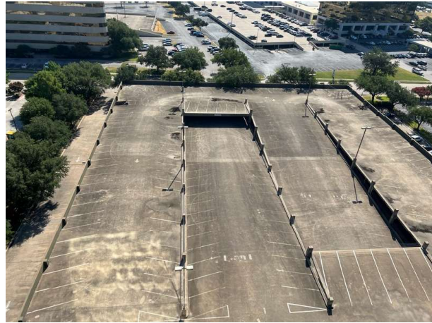
Overall view of parking garage
