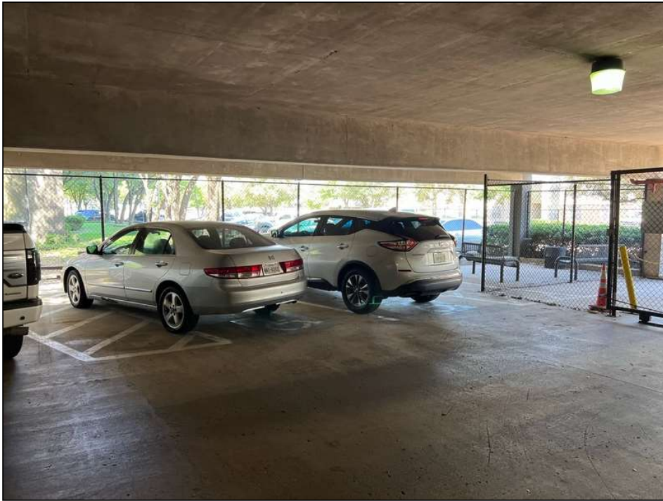
83. Missing accessible parking signs
