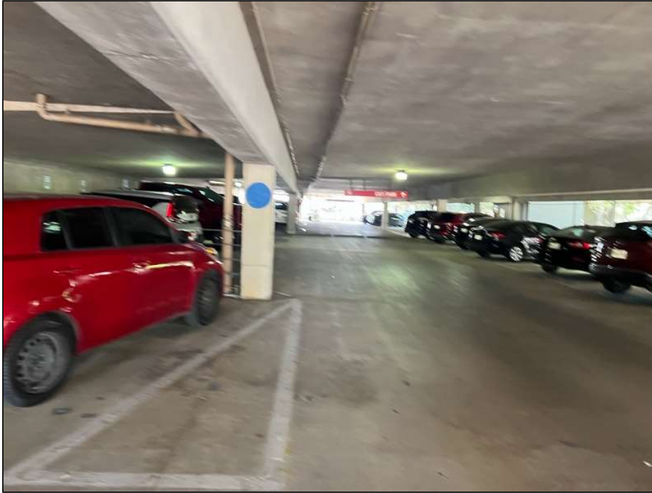
73. Parking garage concrete structure
