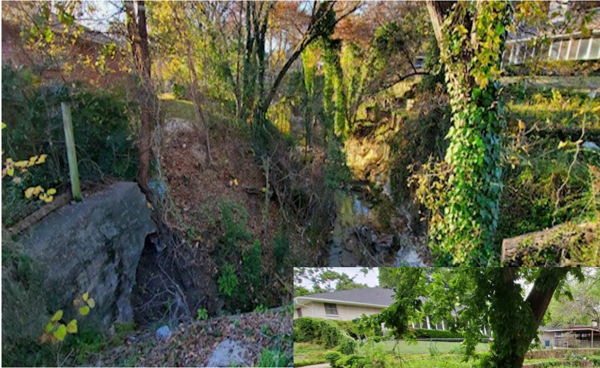
3330/3334 Shady Hollow Ct. Before Construction (2021)
