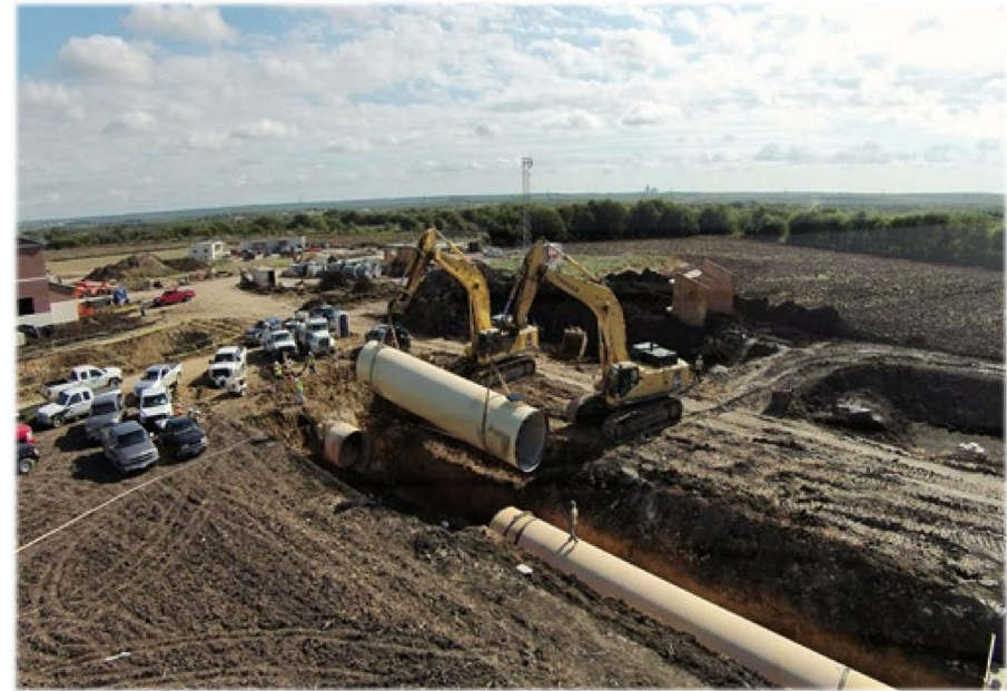
TRWD/ DWU Integrated Pipeline Project
