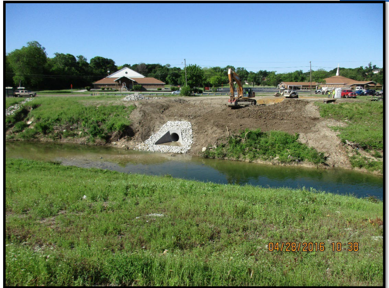
Ledbetter Storm Drainage Project Upsizing a failed 48" Metal Pipe to 60" Reinforced Concrete Pipe (2016)
