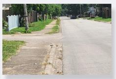
Improvements included the installation of five-foot-wide, four-inch-thick reinforced concrete sidewalks, six-inch-high concrete integral curbs with 18-inch gutters, drive approaches, new slope-downs, and barrier-free ramps.
