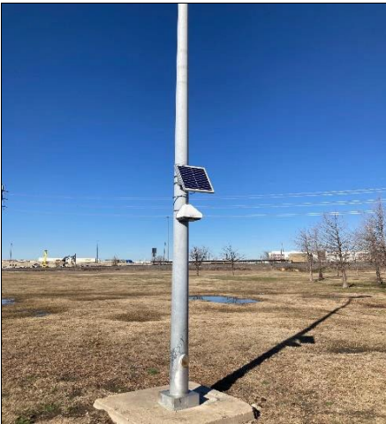
Figure 5. AQ Monitor Installation at Samueli Garland Park (February 13, 2024)
