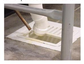
Air Gap - All food contact equipment including food preparation sinks, three compartment sink (if used as food preparation sink), ice bins, and ice machines shall be drained indirectly through an air gap to prevent back siphonage.
