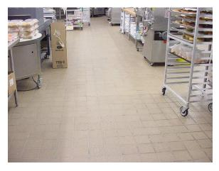
**Floors** - In food/beverage handling and preparation areas, utensil washing areas and restrooms, floors must be constructed of smooth, easily cleanable impervious materials, such as smooth sealed concrete, terrazzo, ceramic, or quarry tile, and graded to trapped floor drains. Wood or absorbent materials are not permitted. Carpet is not recommended in the immediate area adjacent to buffet units. Grouting shall be non-absorbent and impregnated with epoxy, silicone or polyurethane.
