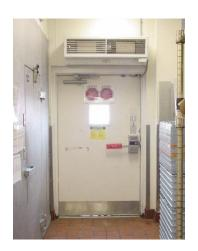
**Exterior Doors and Windows**— All doors leading to the outside must be self-closing and tight fitting, to be effective against the entrance of insects and rodents. Service windows must be self-closing. Service windows may be fitted with 16 mesh screen to meet this requirement.
