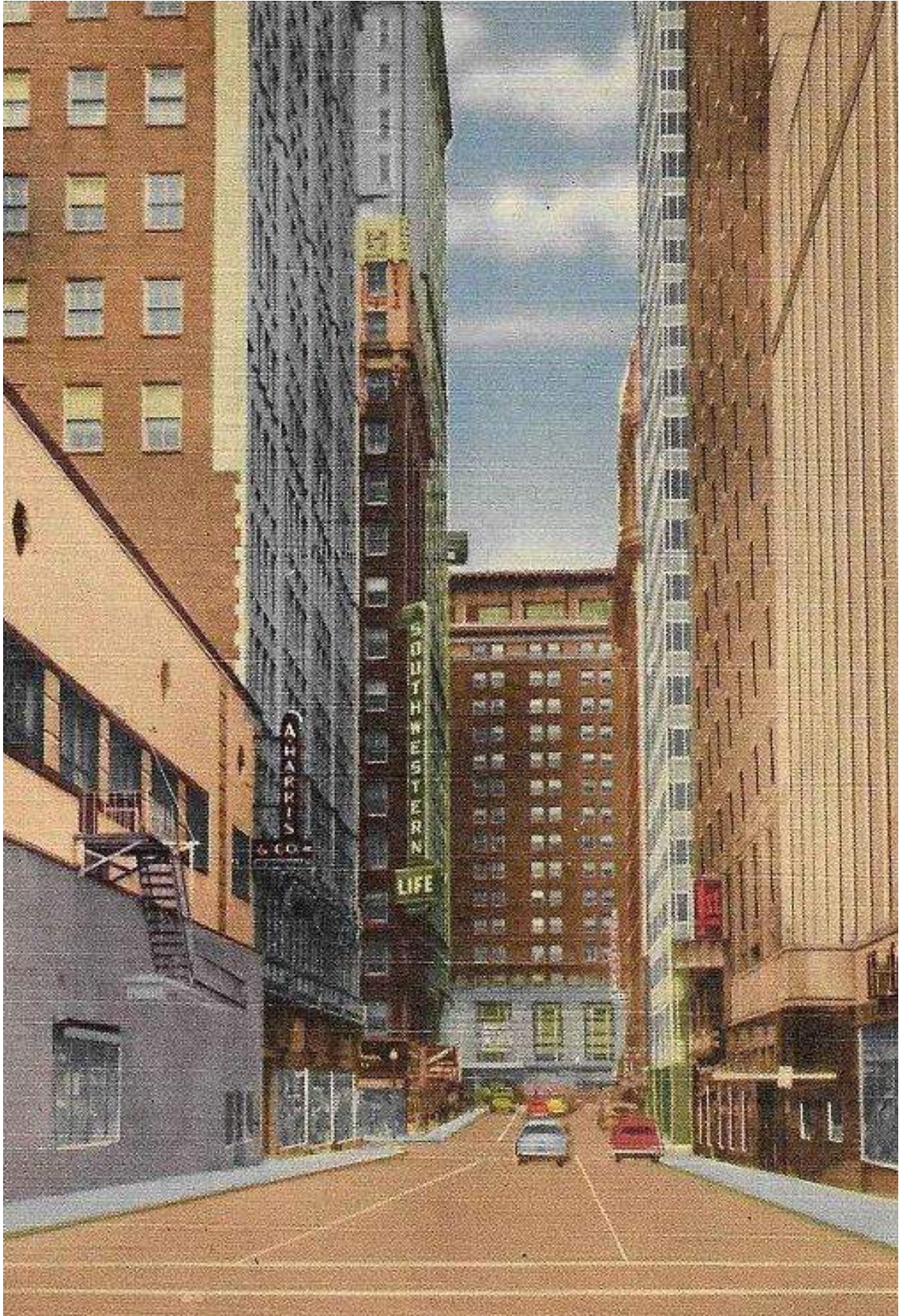
VIEW FROM AKARD LOOKING SOUTH
