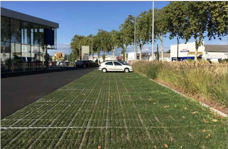
PERMEABLE PAVING AT PARKING AREAS
