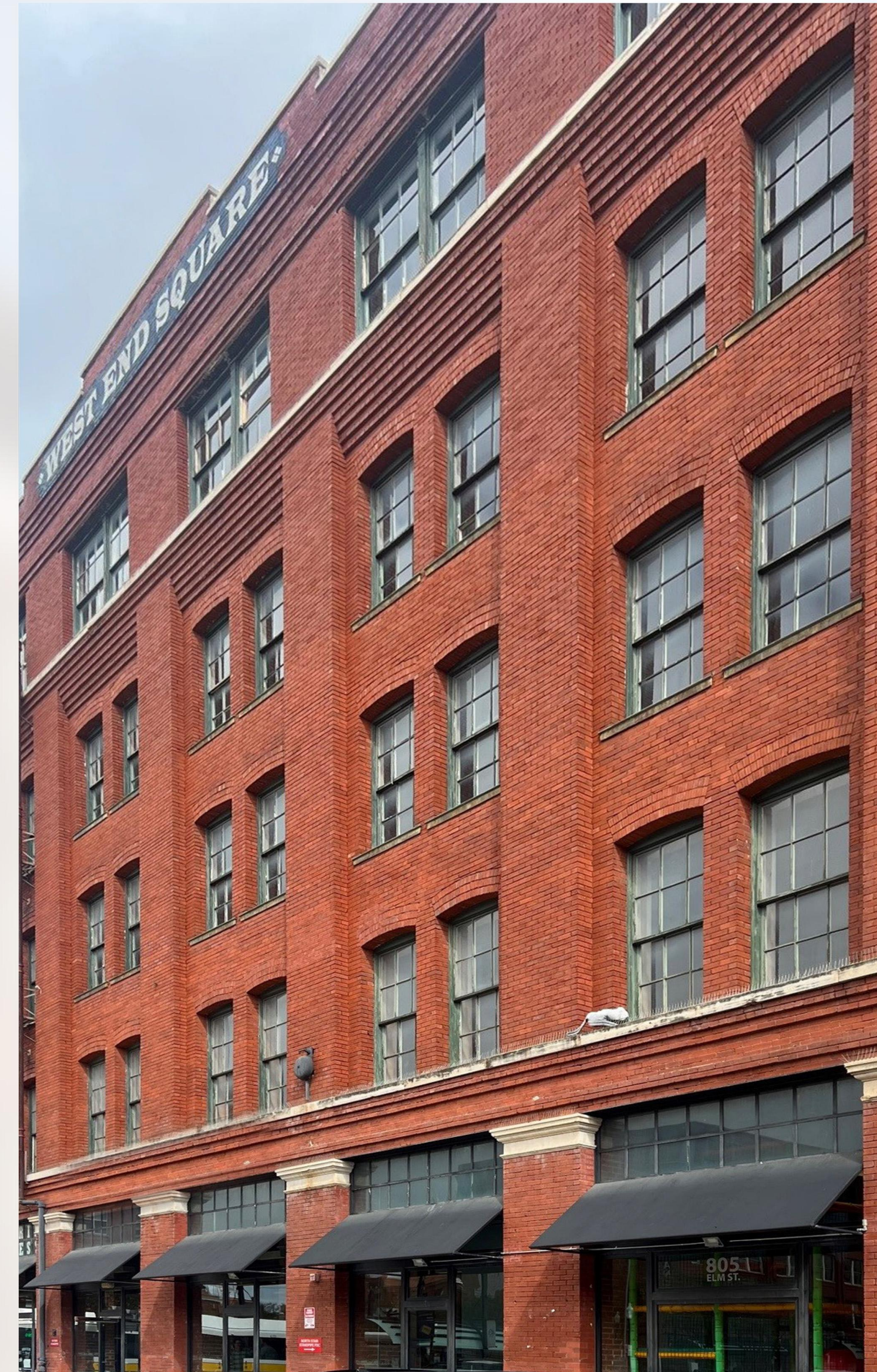
805 Elm Street | Northeast n austin street
