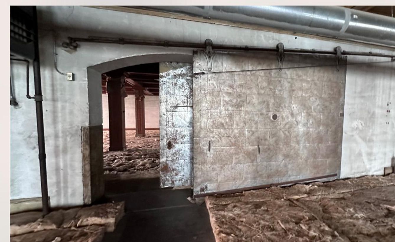
805 Elm Street interior
