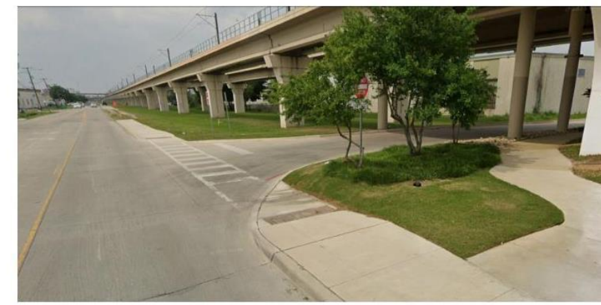
Existing conditions - Denton Drive
