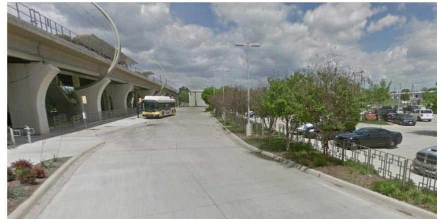
Existing conditions - bus driveway/ parking
