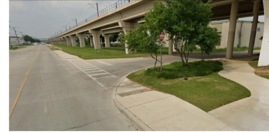
Existing conditions - Denton Drive
