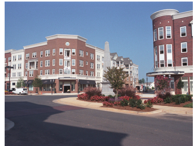
Figure 4.5 (Top) Existing Alvin Street at Garland Road
