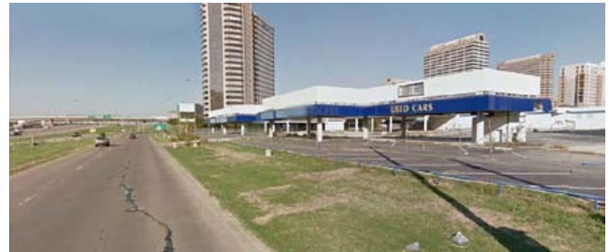
LBJ ACCESS ROAD (EXISTING)
