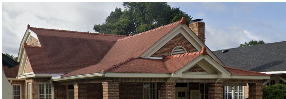
Example: Composition shingles in a color palette of original Spanish tile roofs with terra cotta hips, ridge caps, and rake tiles applied to mimic original tile roofs.
