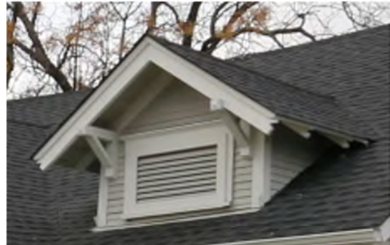
Example: Gabled dormer with louvred vent window.
