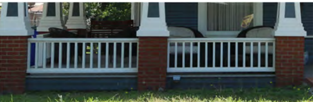
Examples: Wood balustrade on the front porch.
