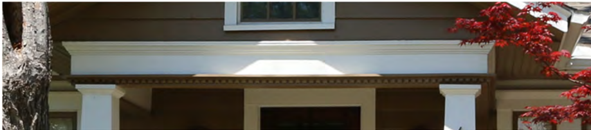
Examples: Minimum 8-inch header beam.
