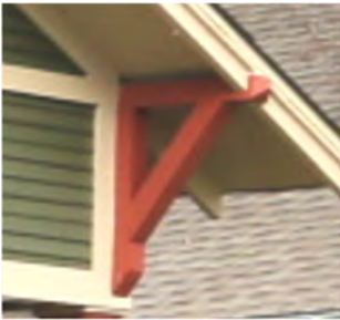
Examples: Decorative roof beams or brackets under gables.
