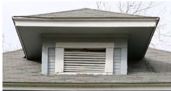
Example: Hipped dormer with louvred vent.
