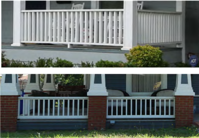
Examples: Wood balustrade on the front porch.
