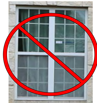
Example: Window grilles behind the glass are not typical of the Transitional Bungalow style.
