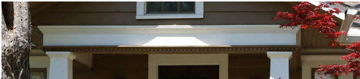
Examples: Minimum 8-inch header beam.
