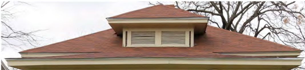
Examples: Centered, hipped dormer with louvered vent.
