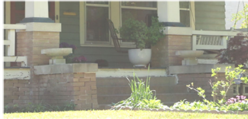
Example: Battered or sloped skirting.
