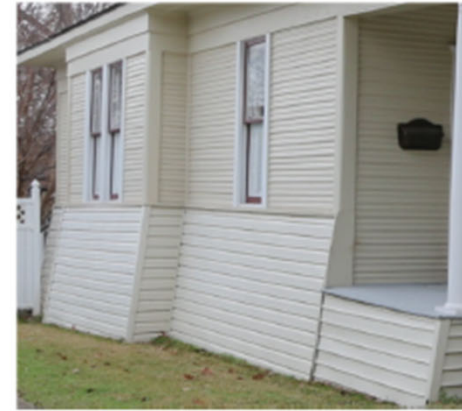
Example: Battered or sloped skirting.
