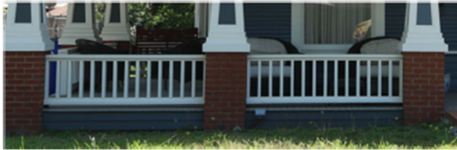
Examples: Wood balustrade on the front porch.
