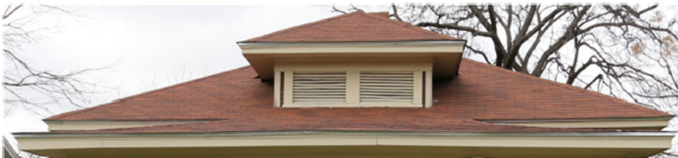
Examples: Centered, hipped dormer with louvered vent.
