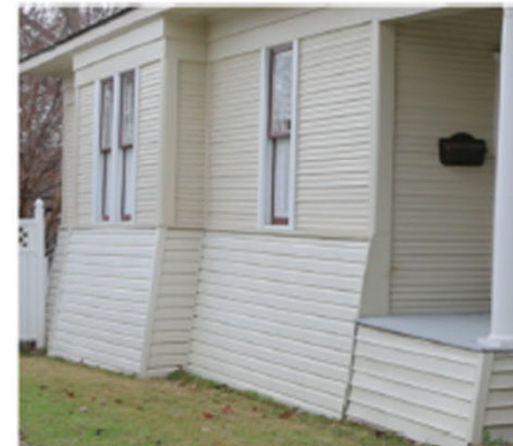
Example: Battered or sloped skirting.
