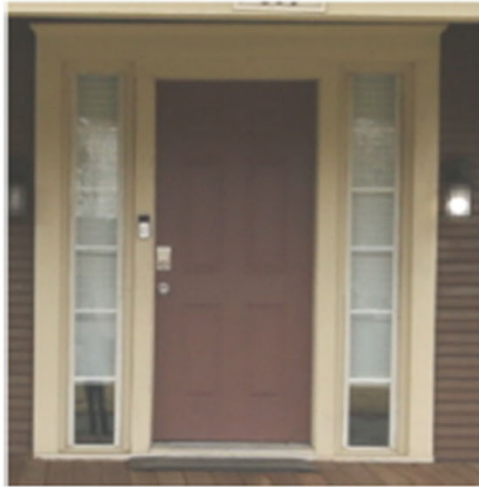
Example: Front door with side lights.
