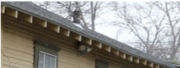
Examples: Exposed rafter tails
