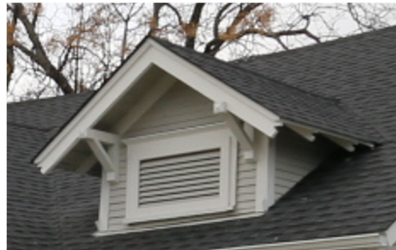
Example: Gabled dormer with louvred vent window.
