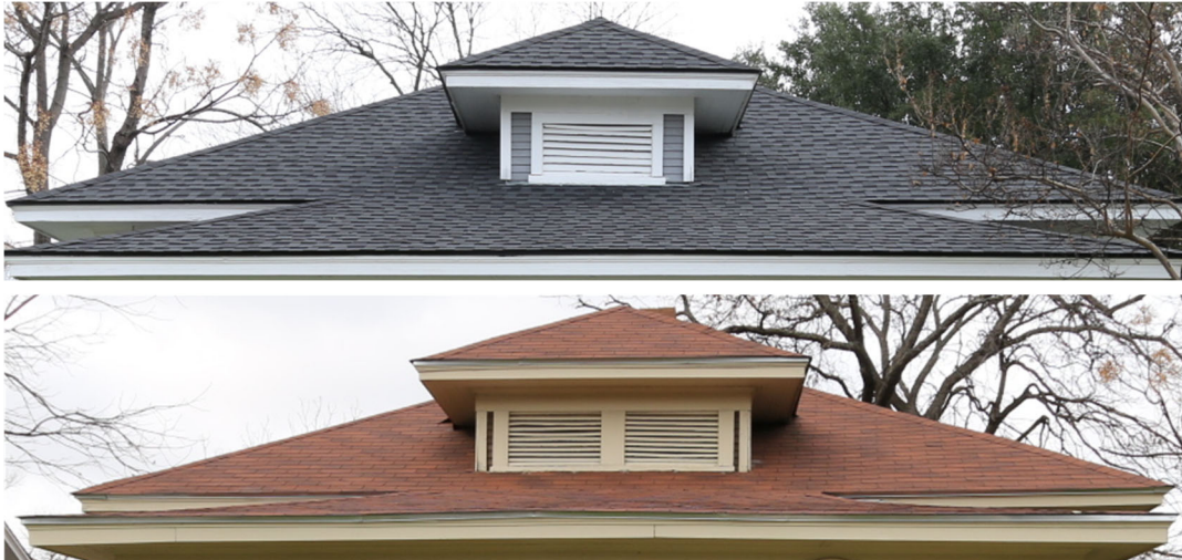
Examples: Centered, hipped dormer with louvered vent.
