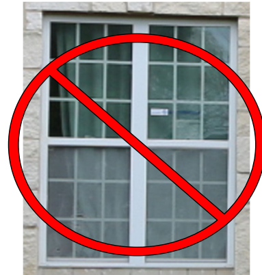
Example: Window grilles behind the glass are not typical of the Craftsman style.
