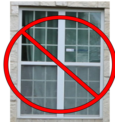
Example: Window grilles behind the glass are not typical of the Transitional Bungalow style.
