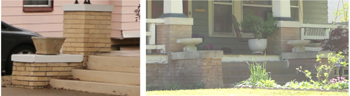
Examples: Wing walls (or cheek wall) on front porch steps.
