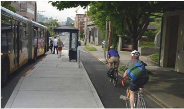
These bike lanes slip behind a train and bus platform, protecting cyclists and providing a buffer to the sidewalk
