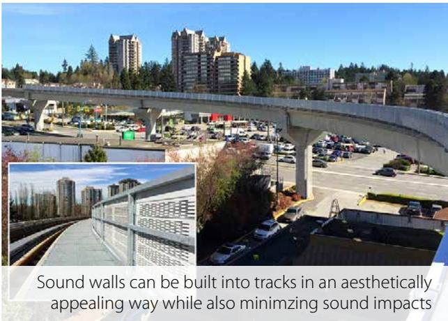
Sound walls can be built into tracks in an aesthetically appealing way while also minimizing sound impacts
