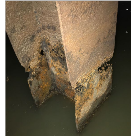
Before and after pictures of columns on Belt Line Road Bridge
