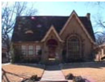
House located in the M Streets East District
