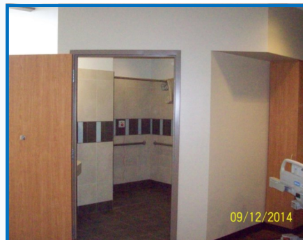
Bathroom at New Parkland patient room
