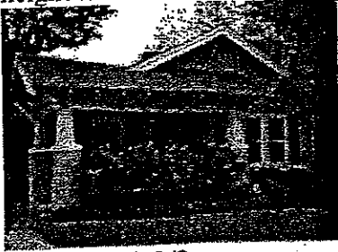
1/3 wood, 2/3 masonry base columns
