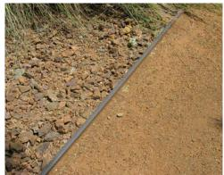
STEEL HEADER AT DECOMPOSED GRANITE **REGIONAL SOURCE** NATURAL STEEL, 1/2" TH
