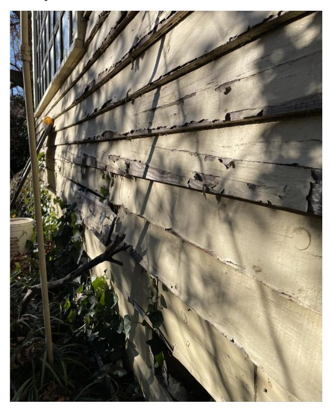
Figure 16 – View of siding showing deterioration of the protective layer of paint and dislodged siding exposing the exterior wall to the elements
