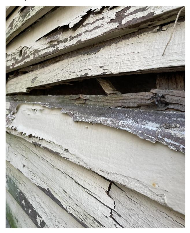
Figure 8 – Close-range view of the wood siding adjacent to a front entrance showing extensive moisture damage and material failure that significantly compromises the integrity of the exterior wall.
