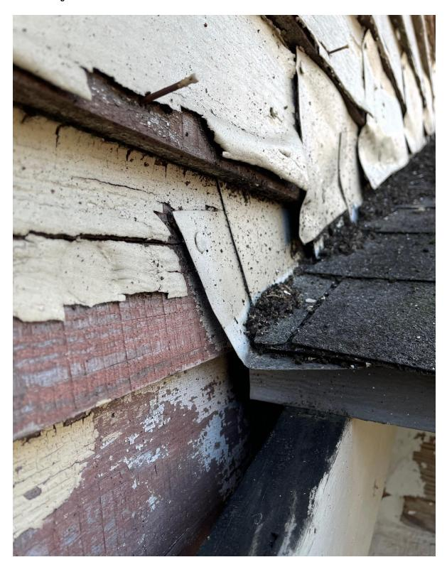
Figure 25 – Detail view of the flashing at the upper wall of the main structure as it interfaces with the lower roof. Ineffective flashing can provide opportunities for water infiltration
