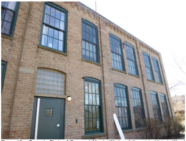
Figure 15 – Example Photo of Proposed Marvin Window Adjacent to Historic Wood Windows; Can you tell which is the replacement?
