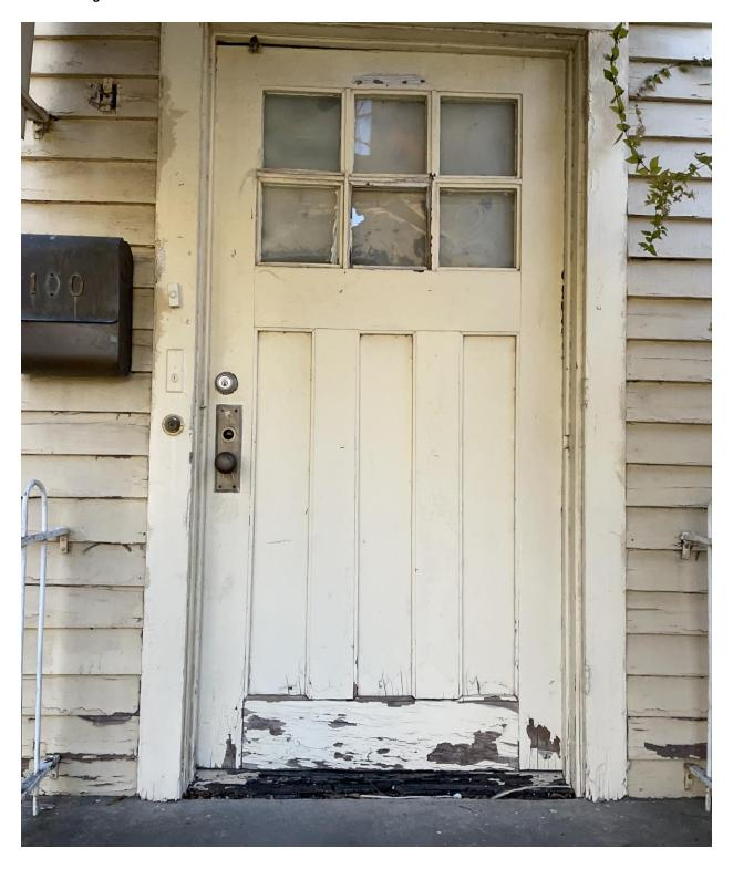
Figure 11 – View of upper level door showing deterioration of the sill
