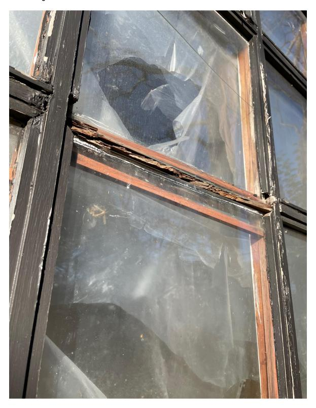
Figure 20 – Detail view of multi-light window showing joint failure and deterioration/loss of the glazing stop, both of which can expose the exterior wall to water infiltration
