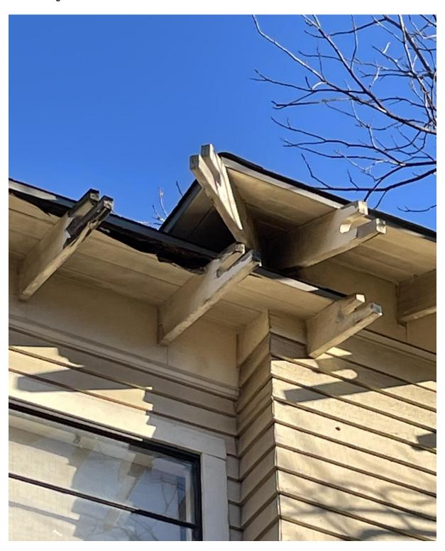
Figure 7 – View of damaged lower soffit and deterioration of the rafter tails facing W  $10^{th}$  Street. Damage such as this compromises the integrity of the roof at an area that is susceptible to water infiltration and also provides opportunities for birds and rodents.
