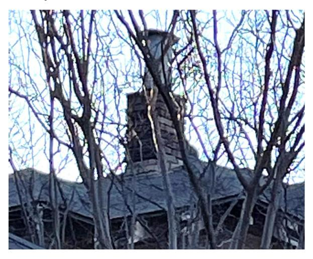
Figure 4 – View of the chimney showing evidence of mortar loss and inadequate flashing
