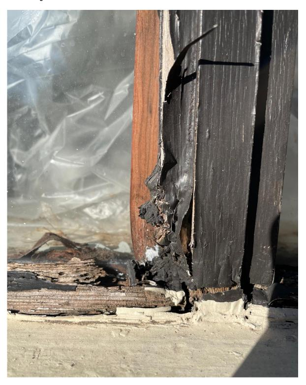
Figure 21 – Detail view of multi-light window jamb at the sill showing material failure, loss of protective coating and deterioration at the sill providing opportunities for water infiltration
