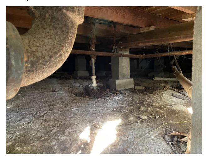
Figure 28 – Partial view of floor structure on concrete posts
