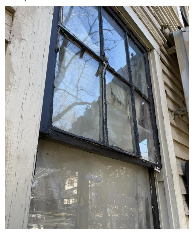
Figure 10 - View of upper sash showing deterioration of the glazing putty, an essential component of weatherproofing
