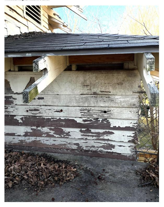
Figure 23 – View of upper wall at exposed rafters showing deteriorating siding, missing siding at the underside of the sloping roof, and drilled holes in the siding all of which provide opportunities for water infiltration and access by birds and rodents
