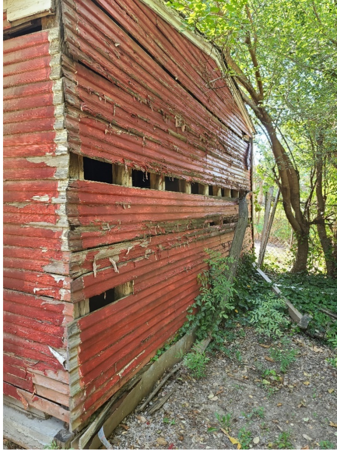
Figure 16 -- Close up of siding on accessory structure.
