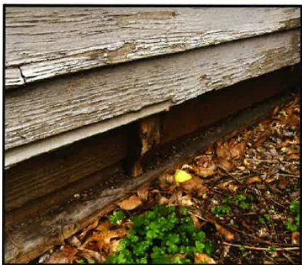
Photo #4: Stud and Sill Plate Rot at North Wall
