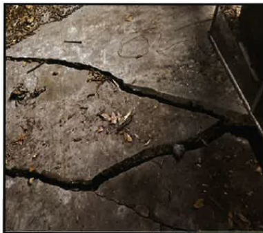
Photo #6: Slab on Grade Crack
