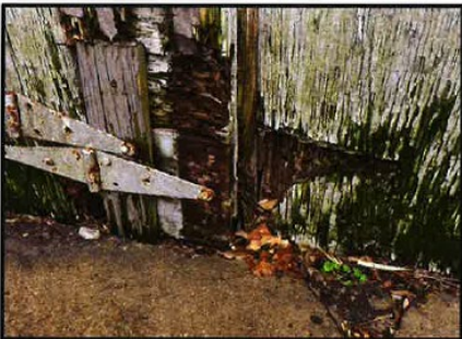
Photo #3: Wood Rot at Garage Doors
