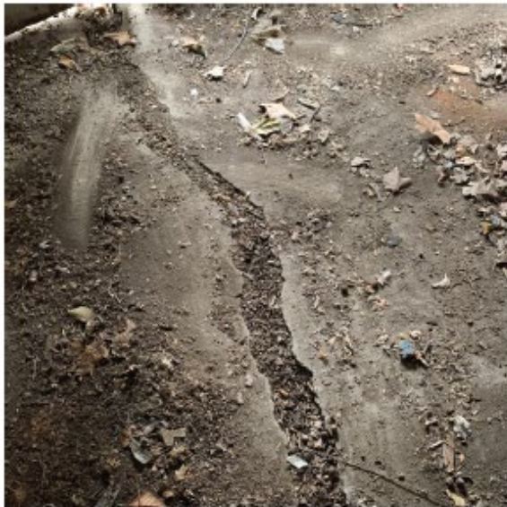
Garage detail for crack running the length of the foundation
