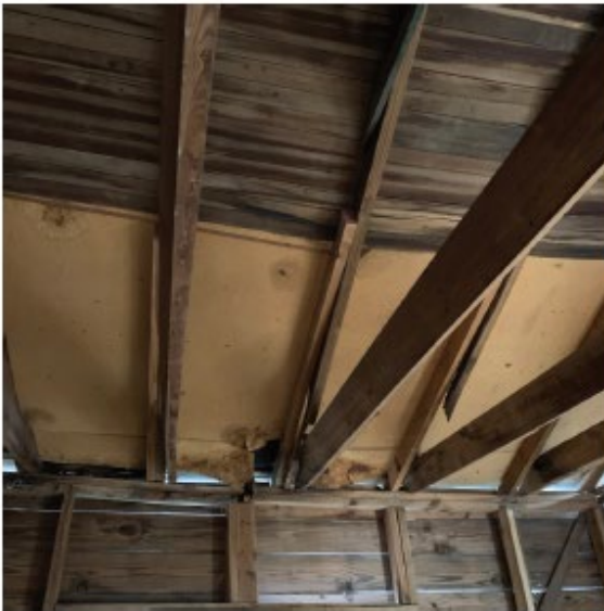
Garage interior south in showing substandard roof repair
