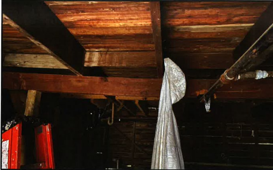
Photo #14: Split and Sagging Support Beam
