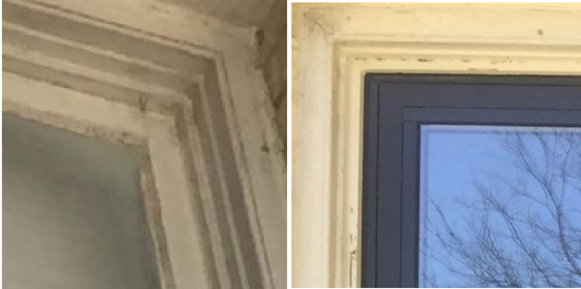
Historic wood window sash vs. vinyl window sash
