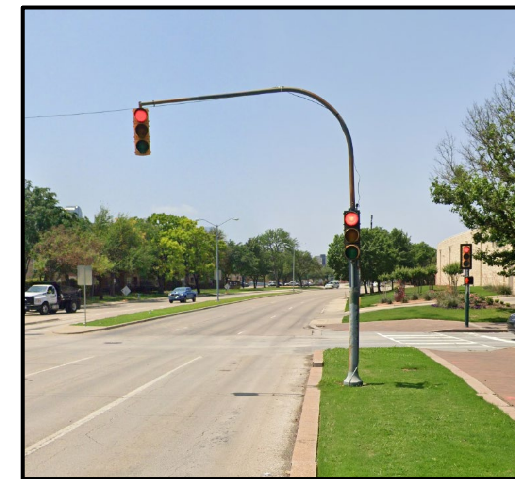
Example of “End of Useful Life” signal infrastructure – outdated mast arm and signal equipment. (Haskell Ave. at Lemmon Ave.)
