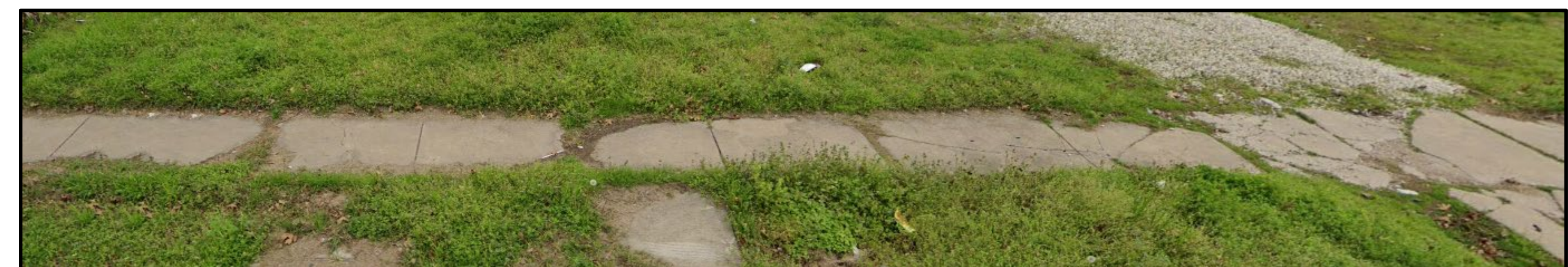
Example of sidewalk in poor condition – deteriorating sidewalk with visual cracking. (Peak St. between Garland Ave. and Ash Ln.)
