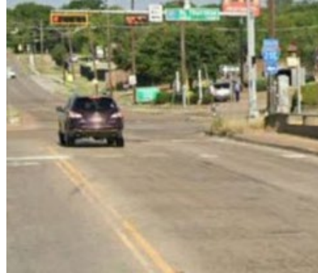
Faded pavement markings
