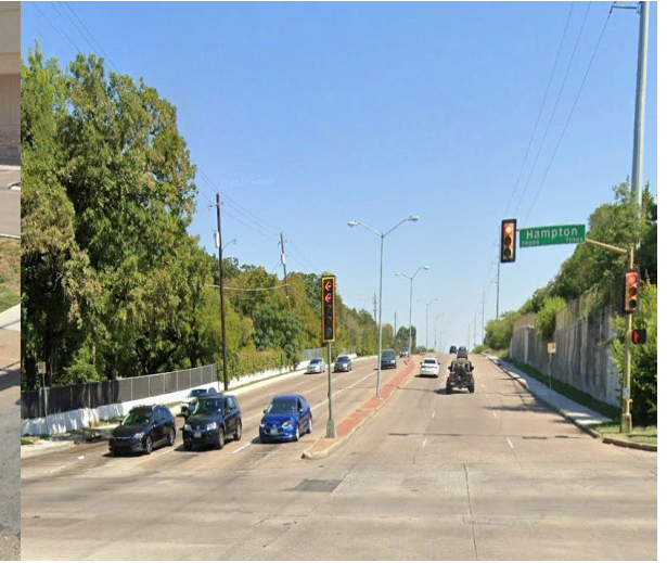
Absence of striped crosswalks at S. Hampton Road
