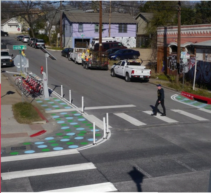
Intersection bumpouts in Austin, Texas.
