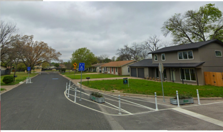
Walnut Hills Dr installation in Austin, Texas.
