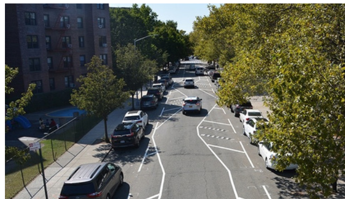
A permanent chicane installed by the New York City Transportation Department
