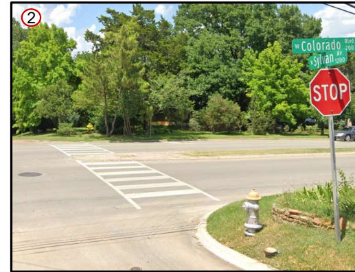
Pedestrian crossing with no controlled pedestrian signal or pedestrian ramps
