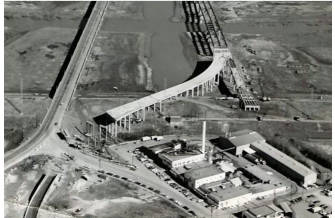
Jefferson Street Viaduct construction is shown on January 11, 1972. The Houston Street Viaduct is at left.
