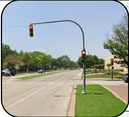
Typical Example of "End of Useful Life" Signal Infrastructure
