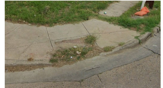
Ramps not ADA compliant
