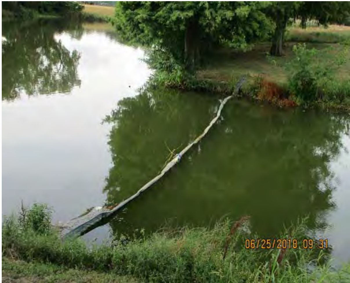
Figure 1-1 Lake Cliff Park Litter Boom
