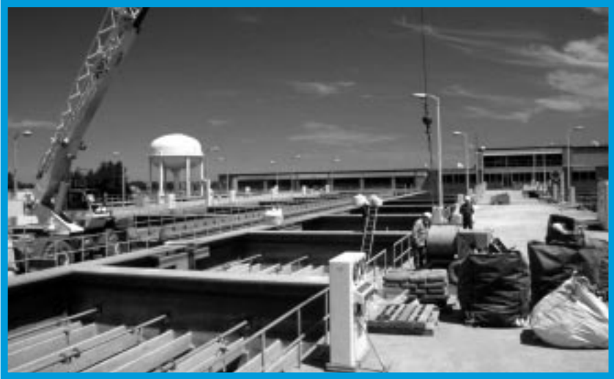
Filters are being rehabilitated at the Eastside Water Treatment Plant.
